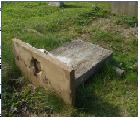
One of the unsafe gravestones in Husthwaite Cemetery
